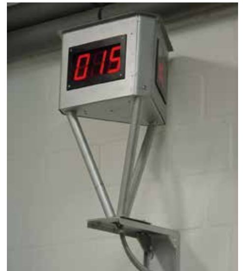
Example: external 3-side temperature display
